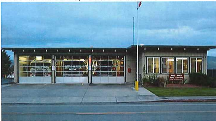
Mad River Station. 3235 Janes Road, Arcata CA 95521
